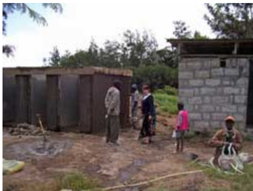
Latrine construction underway
